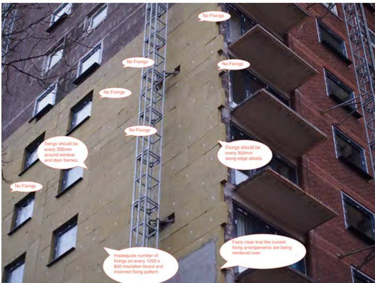
Figure 1. Defects being built into £3m EWI scheme
