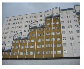
A number of attempts had been made to diagnose the cause of water ingress prior to our involvement. After a detailed site investigation we were able to demonstrate that the metal parapet copings were poorly designed and installed. We highlighted further defects to the external render system caused by a failure to install movement joints.
